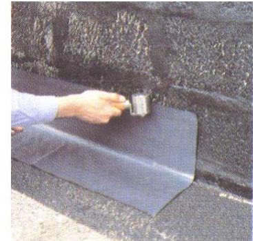
Self adhesive, bituminous waterproofing membranes, used all over the world in extreme climatic conditions, these membranes have become a valid, safe and irreplaceable waterproofing system for 25 years.
